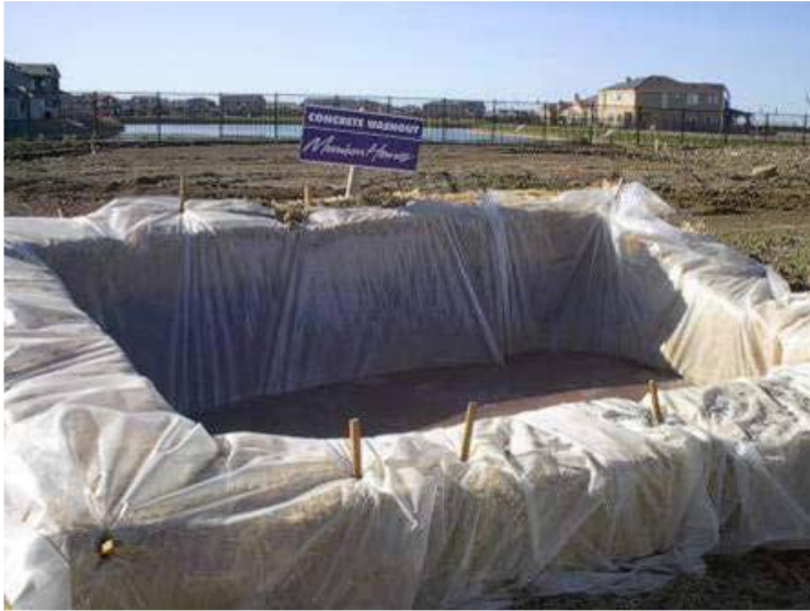
Plate 2.1: Example of a Temporary Concrete Washout Area
